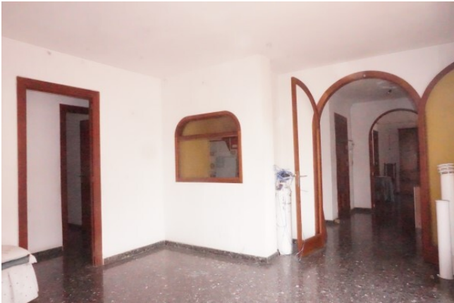
Apartment for renovation
